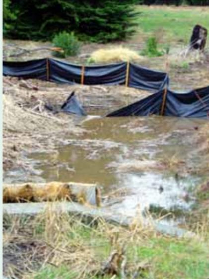
*Channelkeeper documented failing erosion and sediment control measures in a storm in 2007.*
